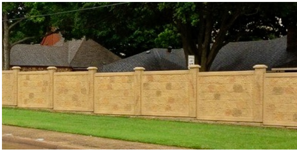
Figure 10. Solid Screening Wall
