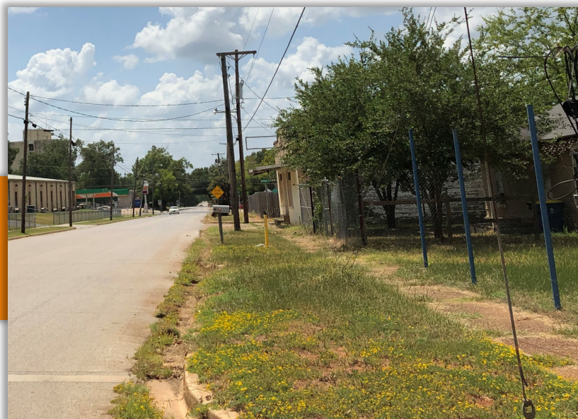
Example of a sidewalk in need of maintenance
